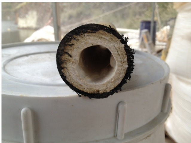
Reagent pipeline blockage due to Gypsum formation.
