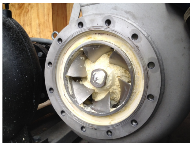
8" pump prior to relocation of reagent input.
